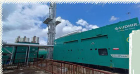
Asset takeover by keolis at depot
