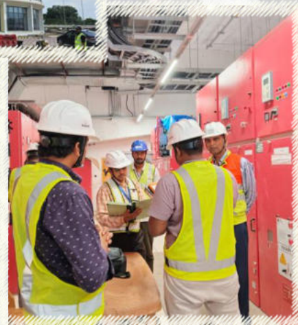
ASS/TSS Room inspection at PMR-10
